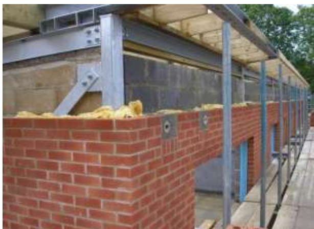
New Barnet, North London: Schwegler "Swift bricks installed in sheltered housing project
